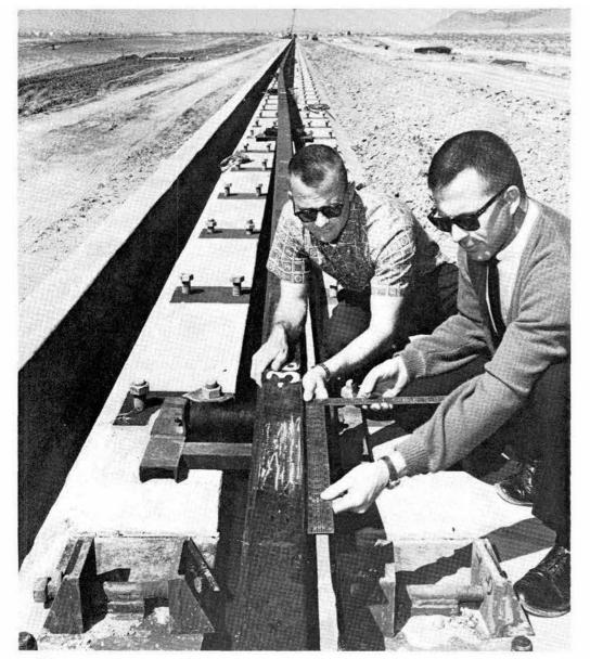
CURVE OF THE RAIL will disappear when the rail is positioned between the bolts of Sandia's new 5,000-ft. sled track in Area III. Inspecting a newly welded rail joint are Bill Kampfe (left) and Marv Timmerman (both 7344). The 39-foot rail sections are welded using a pressure-fusion process and then ground smooth. The new track should be operational in November 1966.
